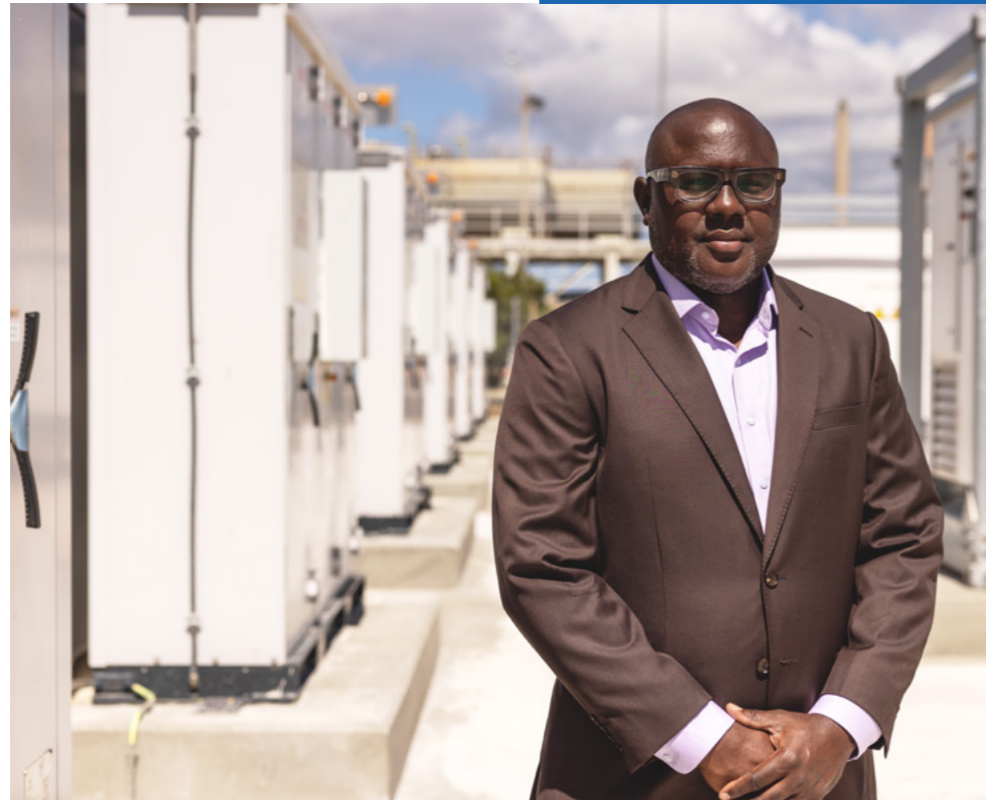
BATTERY ENERGY STORAGE SYSTEM (BESS)
